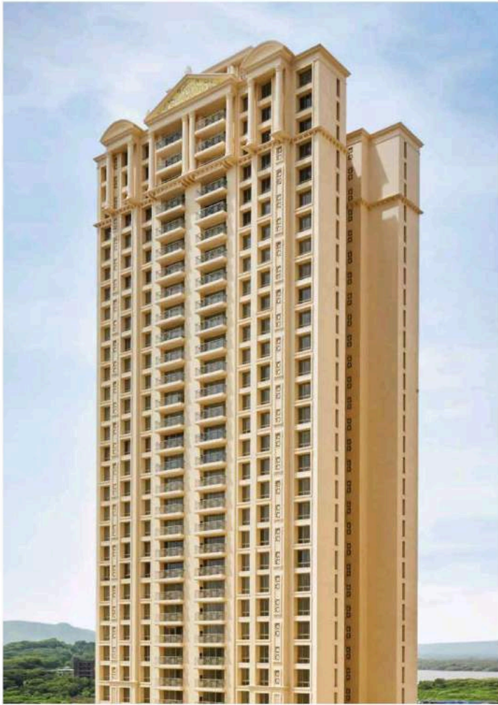
Actual image of Phillipa Building
